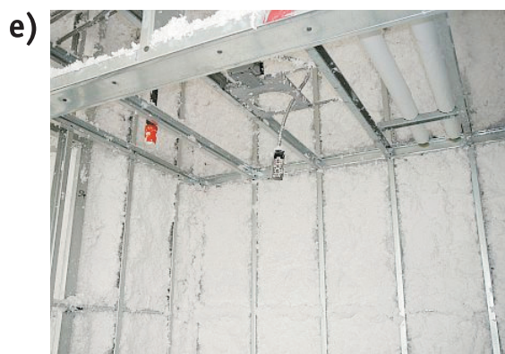
d) Complexity of the framing does not adversely affect the ability to achieve a monolithic installation as illustrated by pictures d) and e).
